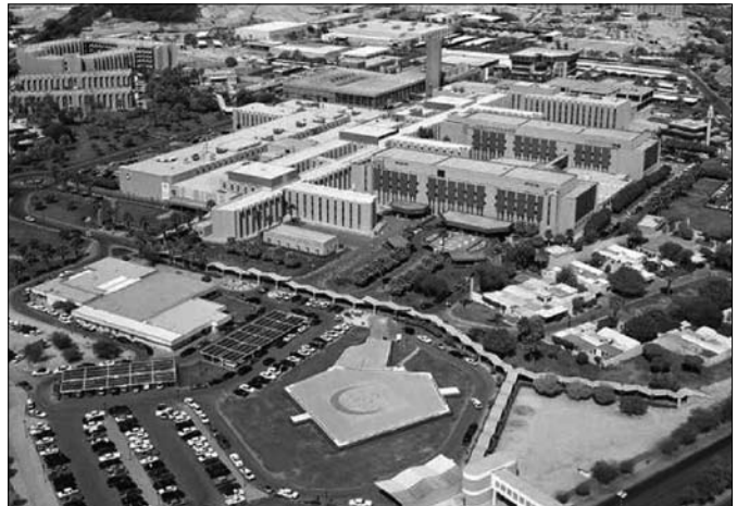
Figure 1. Aerial view of King Faisal Specialist Hospital and Research Centre in Riyadh, Saudi Arabia.
