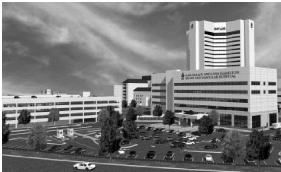
Artist's rendering of the Baylor Jack and Jane Hamilton Heart and Vascular Hospital, scheduled to open in April 2002.
